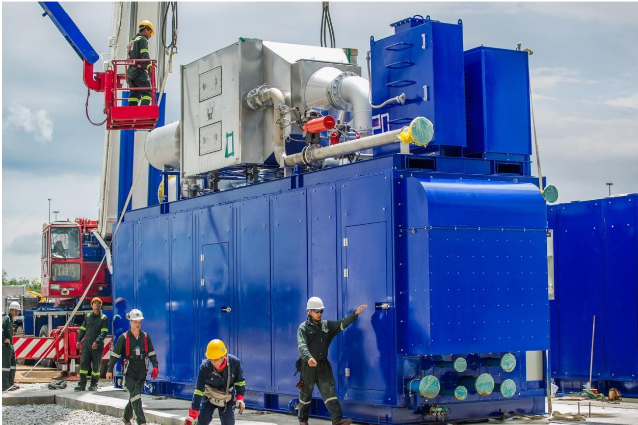
Figure 1. Each Turbophase module is completely self-contained in an 8-ft. x 40-ft. sound attenuated enclosure. A gas-fired engine-compressor set produces compressed air that is added to the combustion turbine's compressor discharge section to reduce the effect of a high ambient temperature or altitude performance derate. Courtesy: Powerphase
